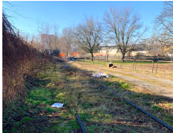
▲ Unmaintained edges along the rail
