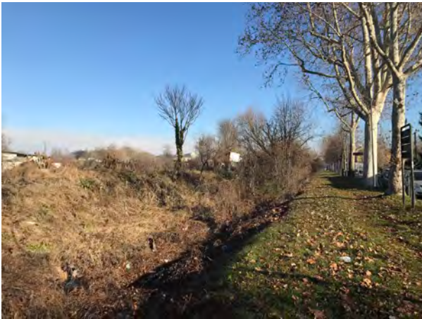
▲ Unmaintained edges along the canal
