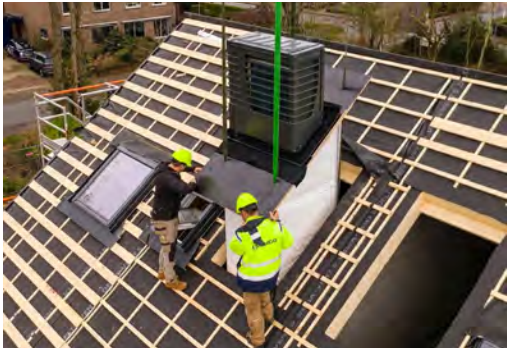
▲ Installing pre-fabricated panels on a roof
