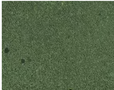
Colored Textured Asphalt
