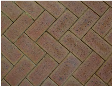
Red Brick Paving
