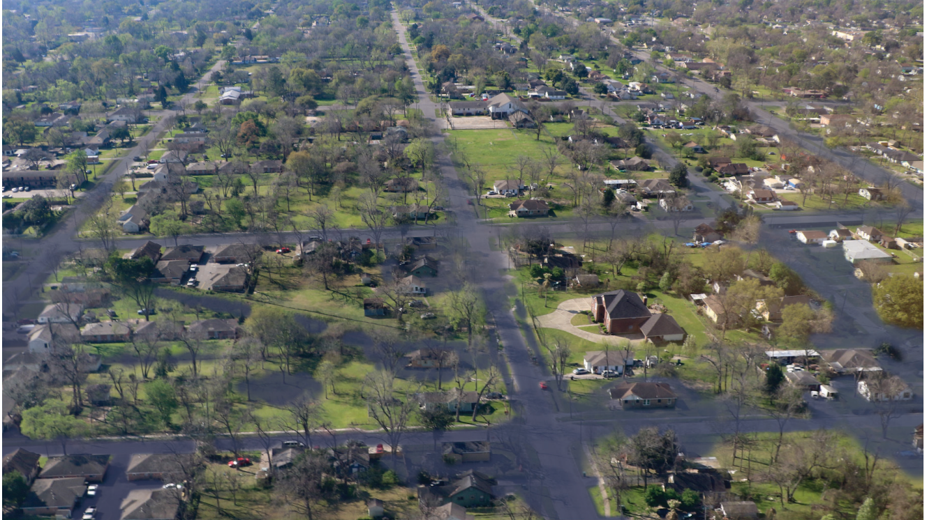
Flooding Before the Introduction of Distributed Detention
